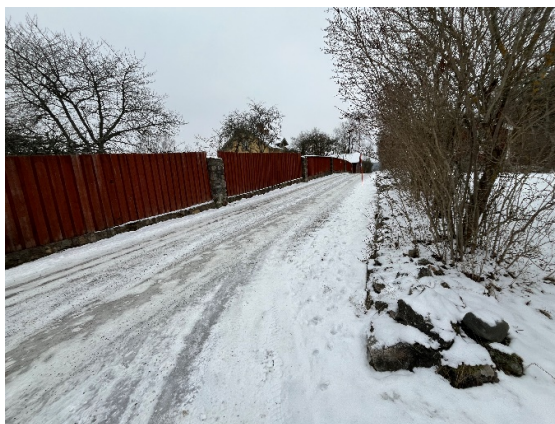
Figur 43 Backa, Vinberga 1:20, mur
